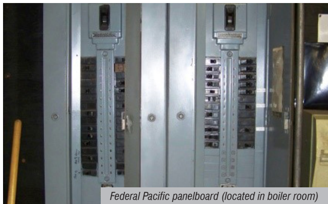
Typical Federal Pacific panelboard installed in the early 1960's
