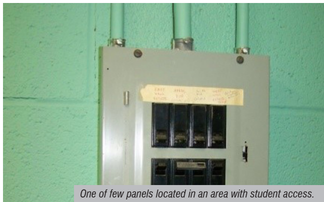
Federal Pacific panelboard (located in boiler room)
