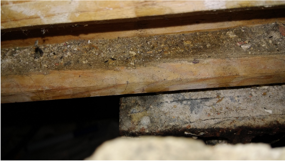
Figure 26 Tongue and Groove over I-Beam Room 305
