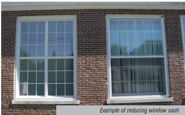
Typical double hung window
