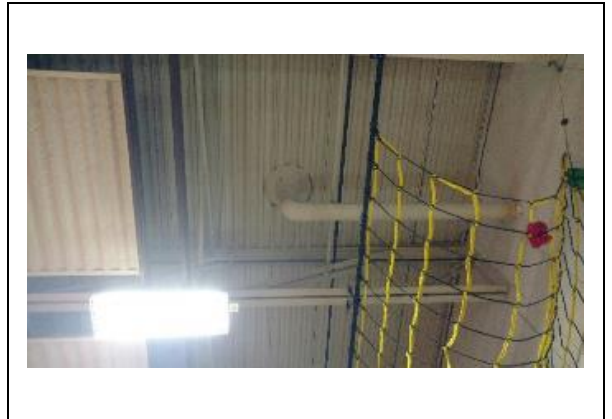
14. Assumed ACB roof drain at Main Dunstable.
