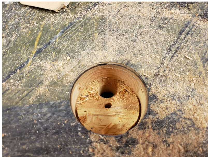
Figure 2 Wood Bore Hole
