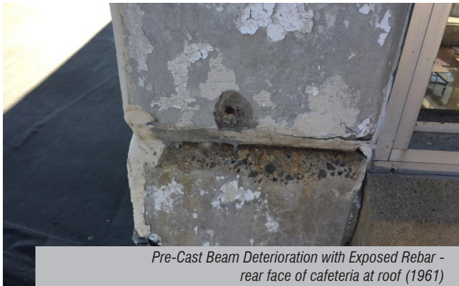
Pre-Cast Beam Deterioration - rear face of cafeteria at roof (1961)
