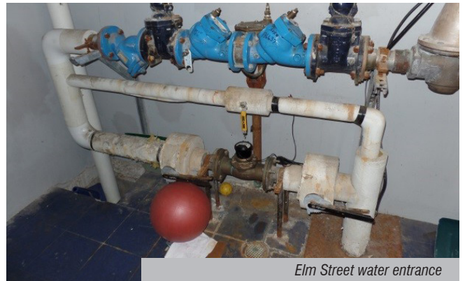
Transition to site piping with no insulation
