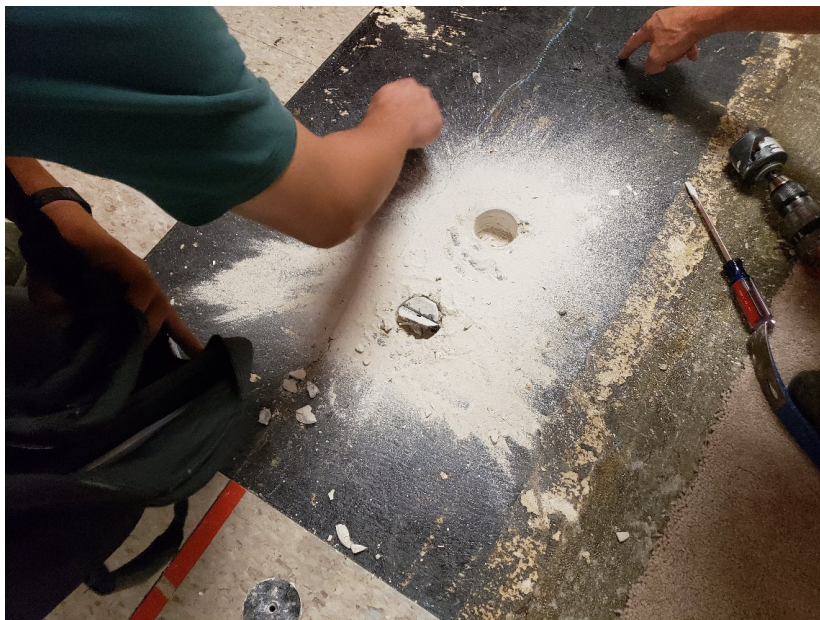
Figure 4 Gypsum Panel Bore hole
