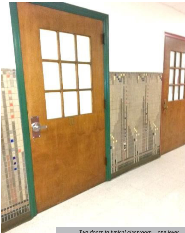
Two doors to typical classroom – one lever handle and the other original knob
