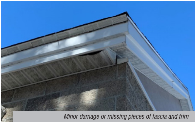
Minor damage or missing pieces of fascia and trim
