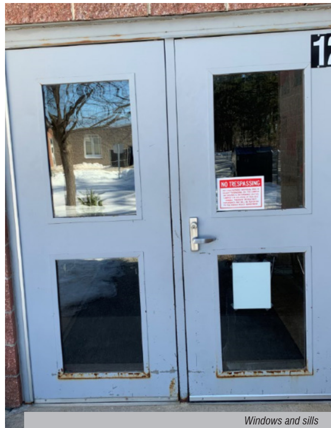
Windows and sills
