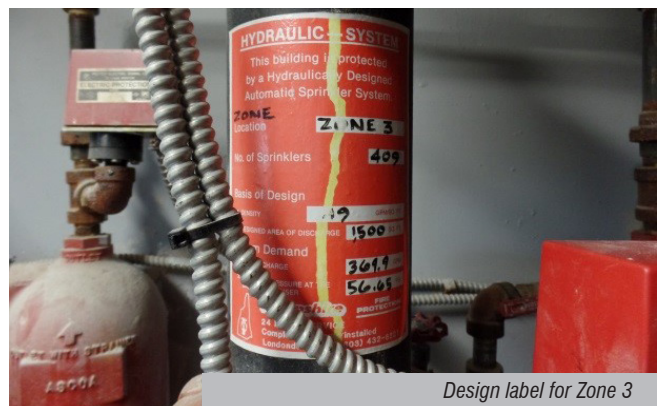
Alarm valve riser #3
