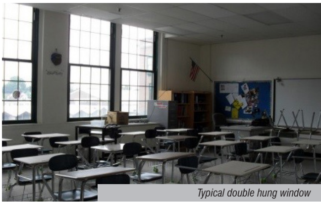
Typical double hung window
