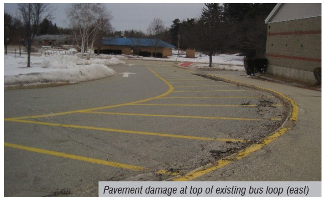
Potholes and pavement in general disrepair
