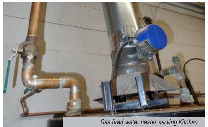
Main Boiler Room gas fired water heater
