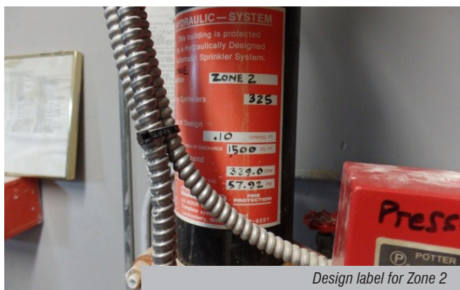
Alarm valve riser #2
