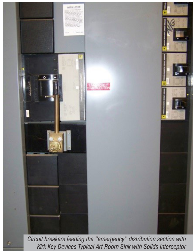
Main Distribution Switchboard - MDP
