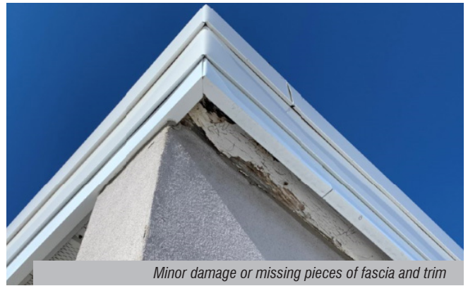
EIFS (exterior insulated finish system) damage/painting
