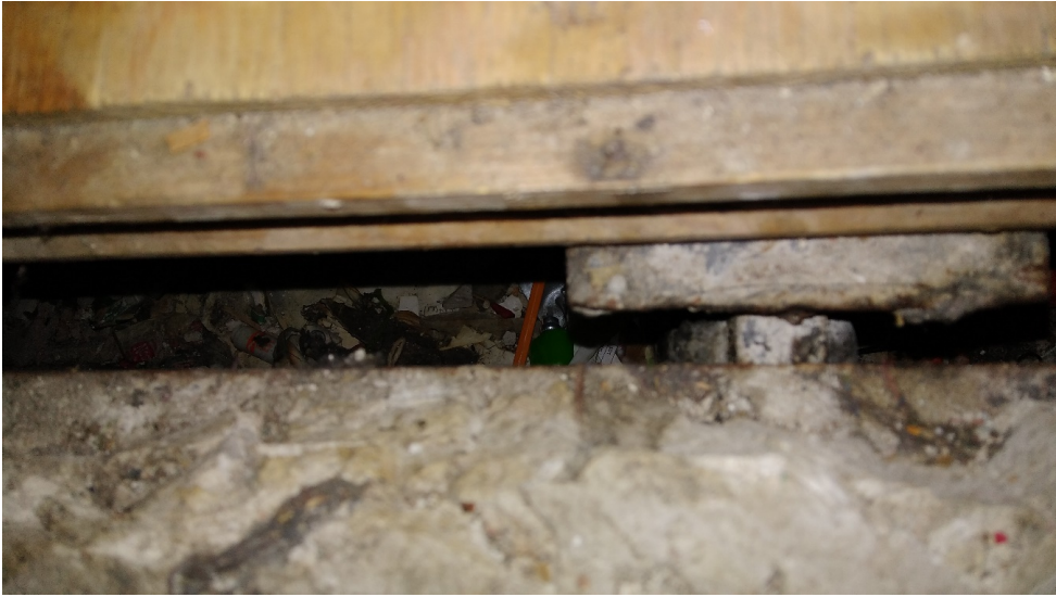
Figure 27 Tongue and Groove over I-Beam Room 305
